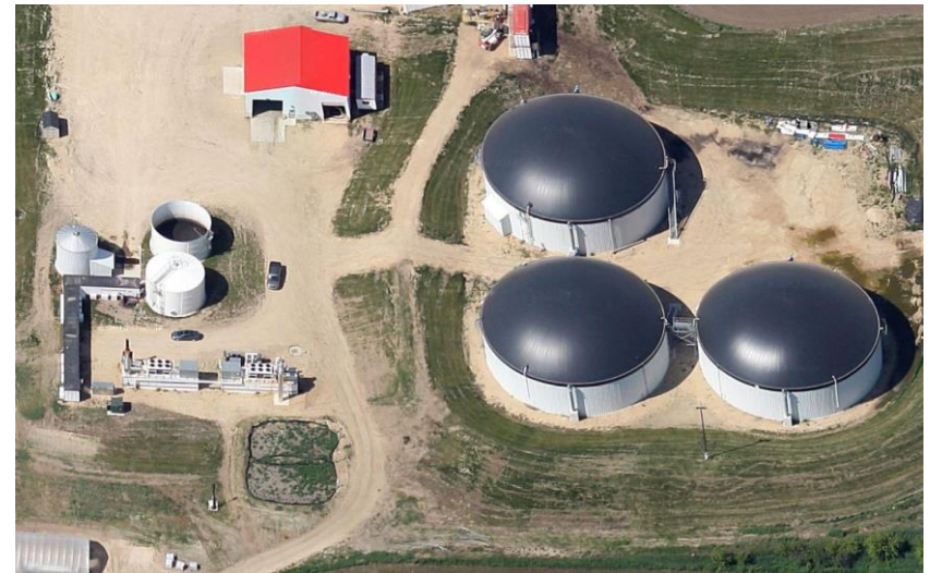
Dane County Community Digester
